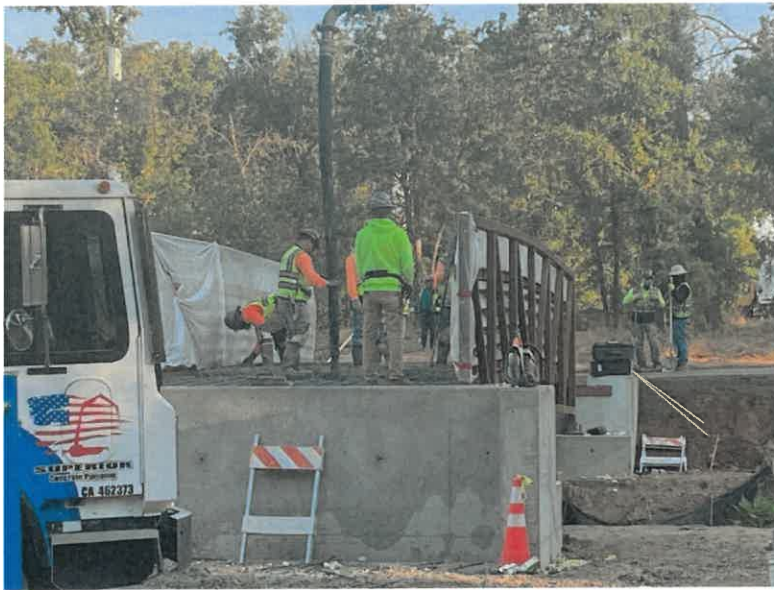
Pouring the bridge concrete floor (10/20/23)
