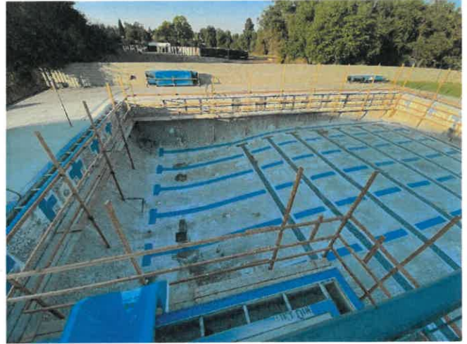
10/18/23 Lane Line & Target Tile Installation
