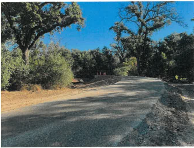
Ramp leading to the bridge (10/29/23)
