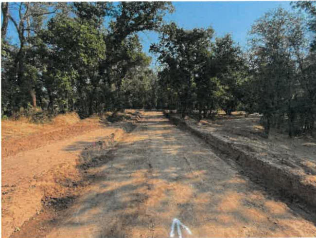
Trail to the east of the bridge (10/18/23)
