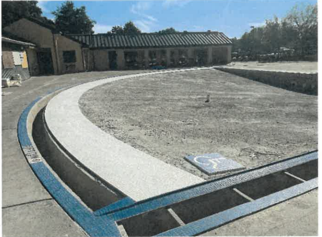
10/20/23 Pool Entry Tile Installation
