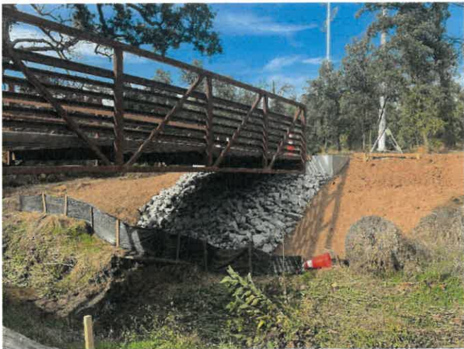
Same view with the added rip-rap and graded soil (11/4/23)
