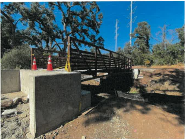
Looking under the bridge (10/23/23)
