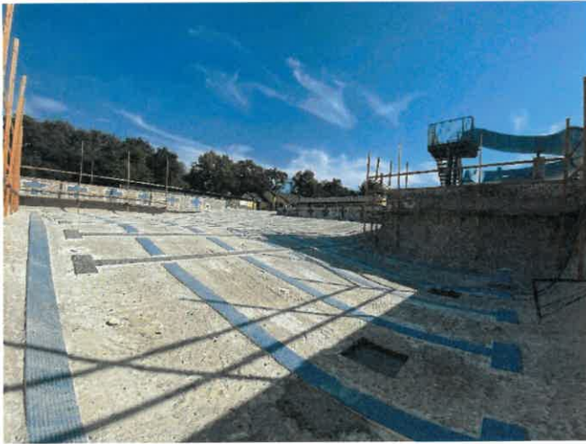
10/20/23 Lane Line & Target Tile Installation
