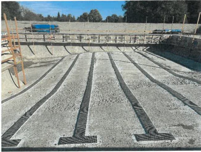
10/13/23 Lane Line & Target Tile Installation
