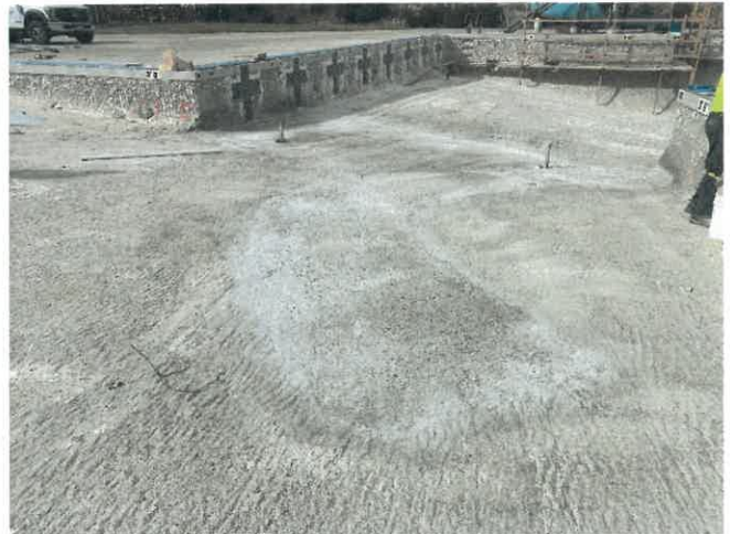
10/10/23 Repaired Cracked Area of Pool
