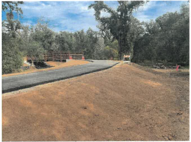
Graded soil along the ramp (11/4/23)
