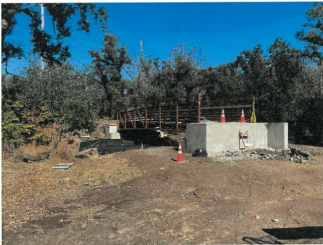
West bridge abutment before the ramp (10/23/23)
