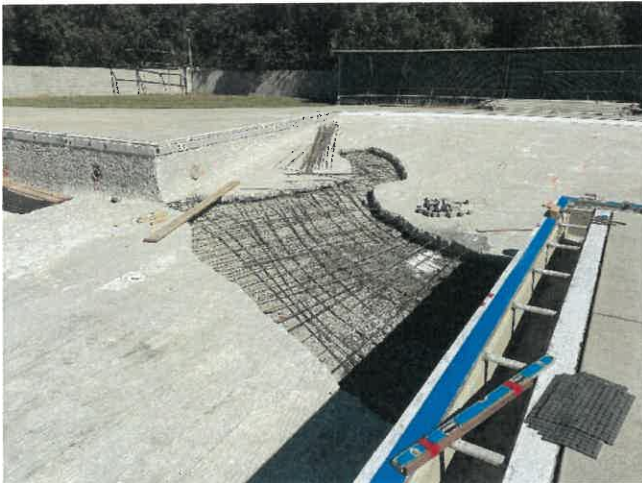
10/5/23 Repairing Cracked Area of Pool
