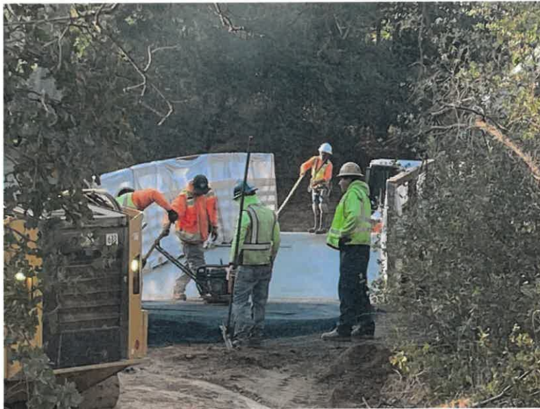
Smoothing the concrete floor and blending with asphalt trail (10/20/23)
