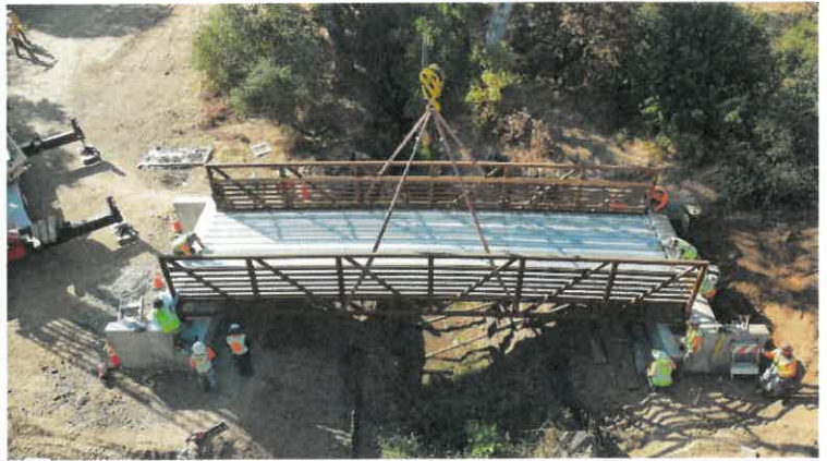
Bridge being set in place (10/19/23)
