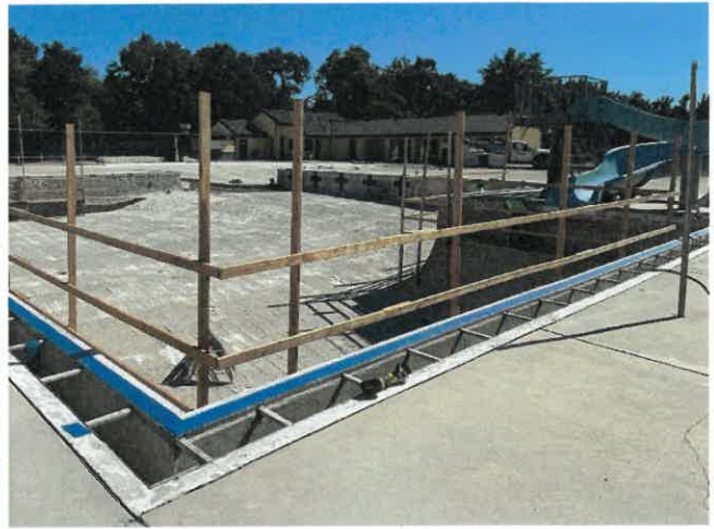
10/5/23 Gutter Tile Installation
