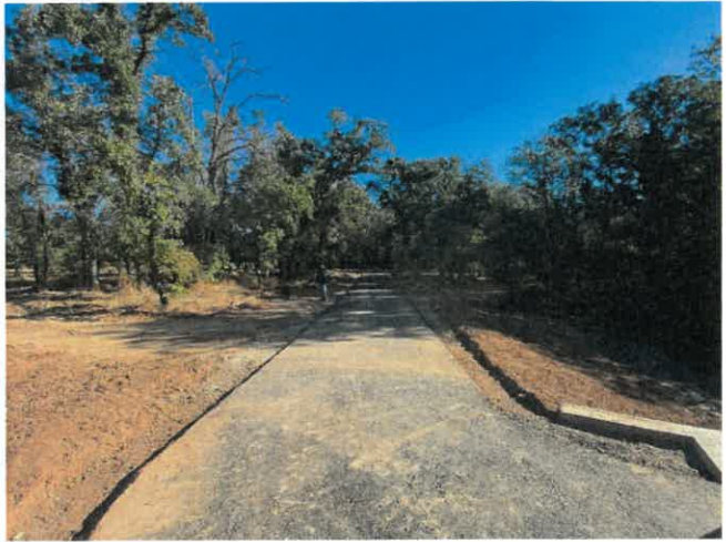
Trail to the east of the bridge (10/29/23)
