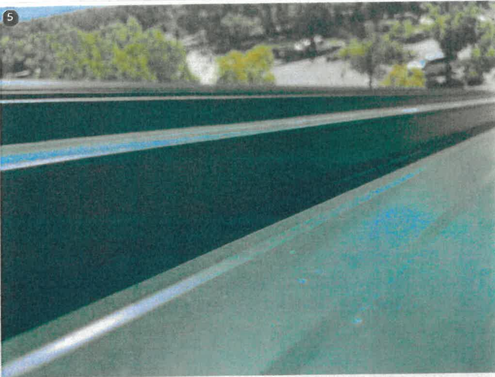
5 Upclose of the ridge cap installed and sealed.
