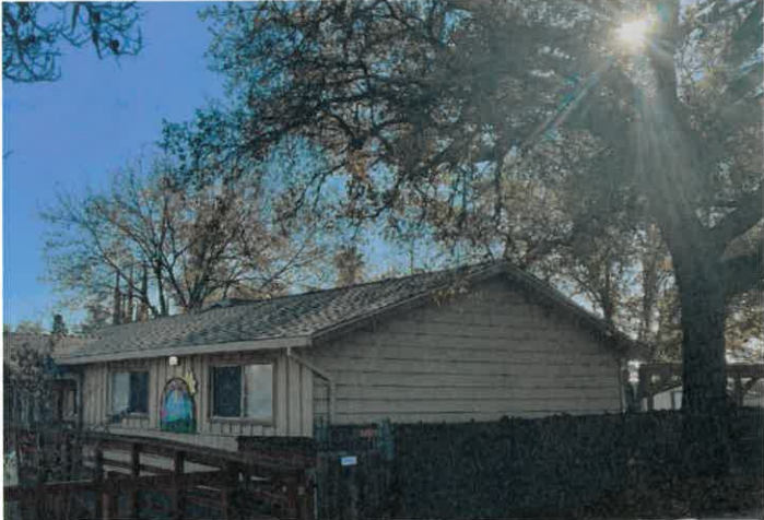
New roof on the Kidz Korner Preschool
