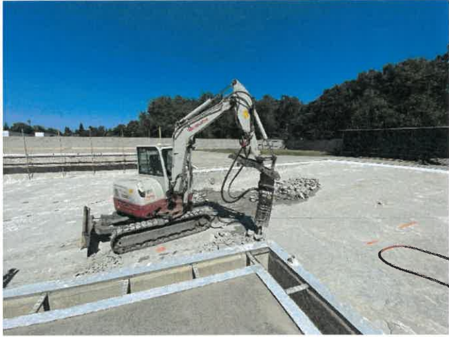
9/28/23 All Tile is Removed & Opening Crack Area
