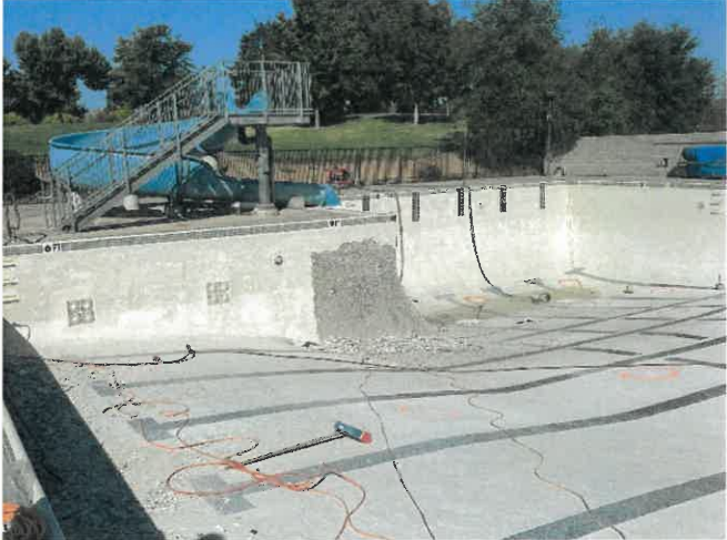
9/19/23 Begin to Remove Plaster
