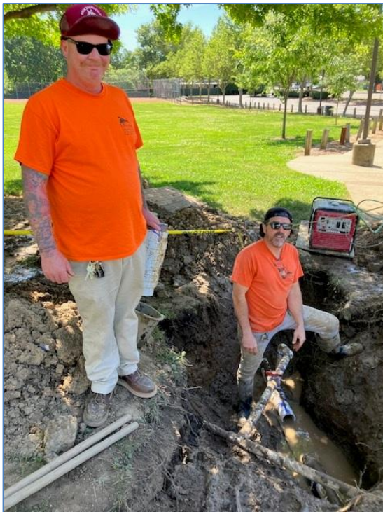
Parks Team Repairing Main-line
